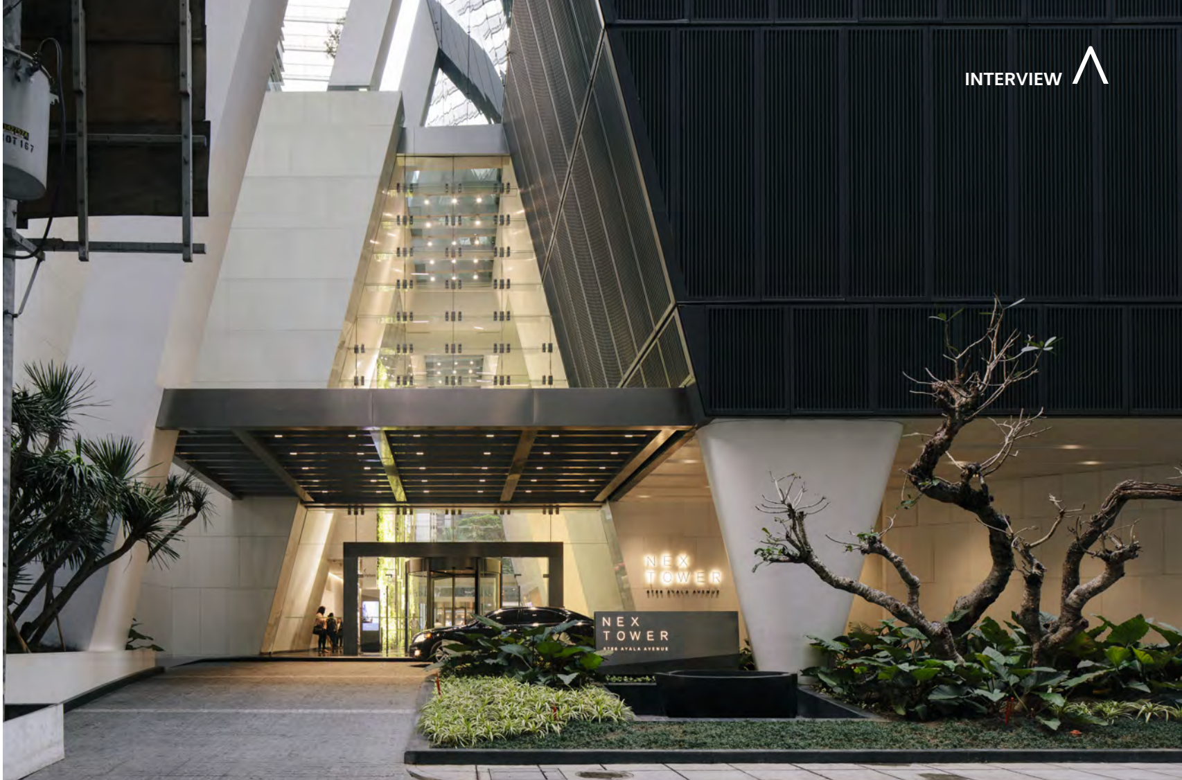
NEX Tower in Manila – a project by SOM. Photo: © Studio Periphery
